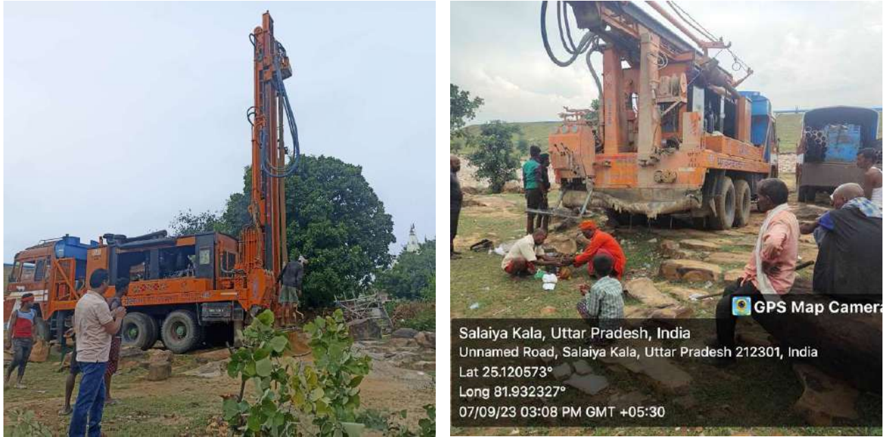
Figure 6.5: Drilling operation in progress for construction of the Piezometer around new Ash Dyke, NTPC Meja,
