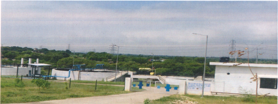
Fig: STP in township area
