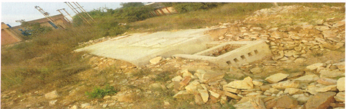
Fig: Rainwater harvesting structure: Township
