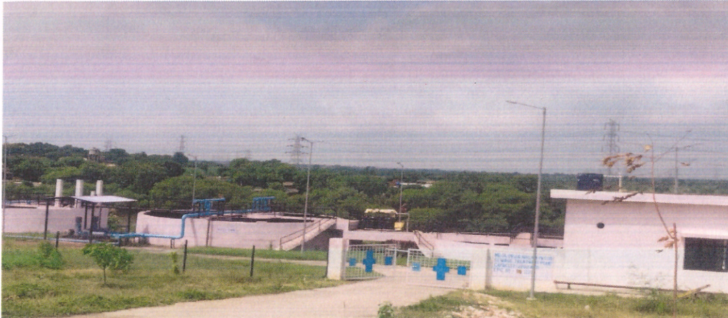
Fig: STP in township area
